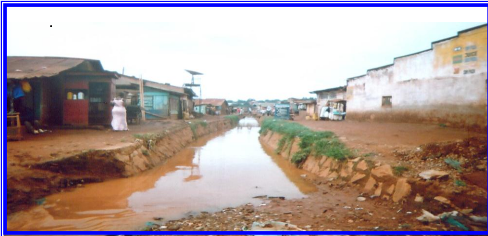
Plate 1: Blockage by silt, garbage and sediments in the Nakamiiro Channel in Bwaise II Parish.
