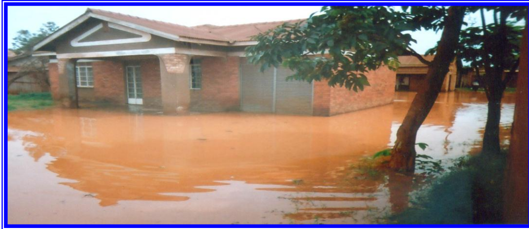
Plate 4: Effects of poor drainage on the quality of living in Bwaise II Parish whenever it floods.
